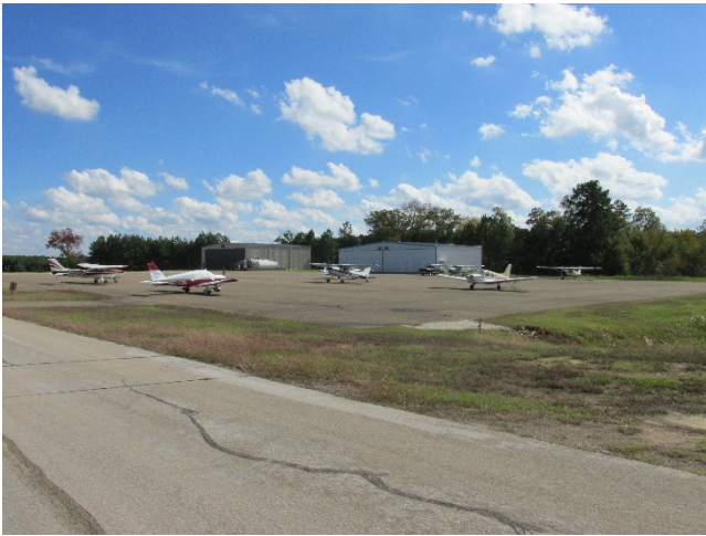
Aircraft Apron and Executive Box Hangars
