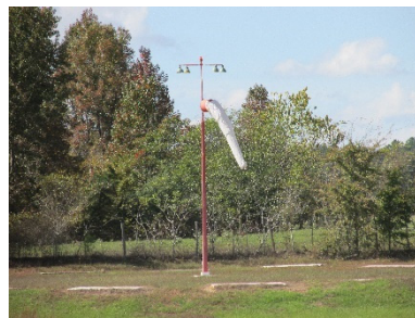
Segmented Circle and Lighted Windcone
