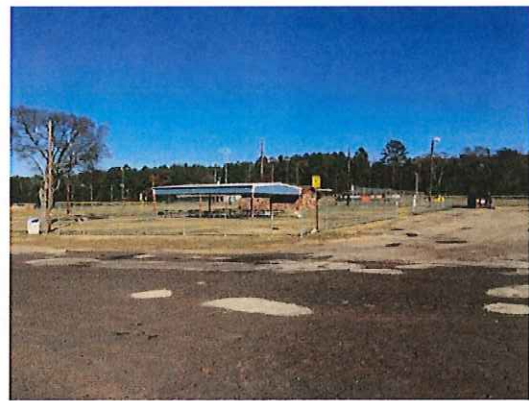
Pavilion and Parking
